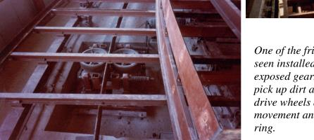
One of the friction wheel drives can be seen installed in its pit. There are no exposed gears, or lubricating grease to pick up dirt and contamination. The drive wheels are free to float with radial movement and are centered by the drive ring
